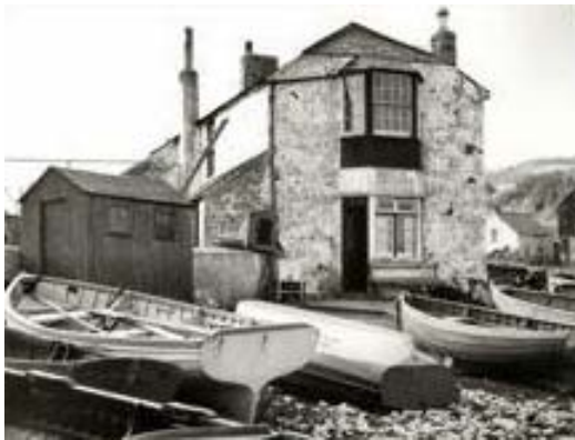
The 1820s watch house at Portmuck, Co. Antrim, where the boat door has been replaced by a canted bay.
